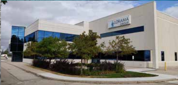
Lorama Group Manufacturing Facility, Canada
